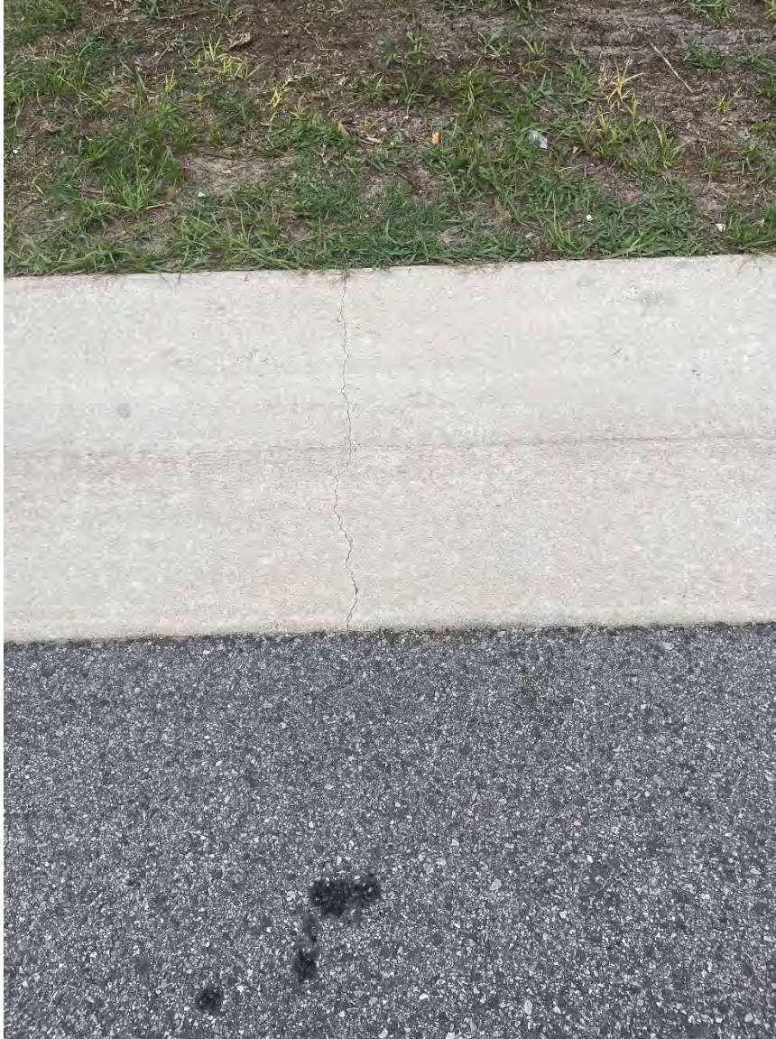
Gutter crack across between 13611 and 13603 Seabridge
