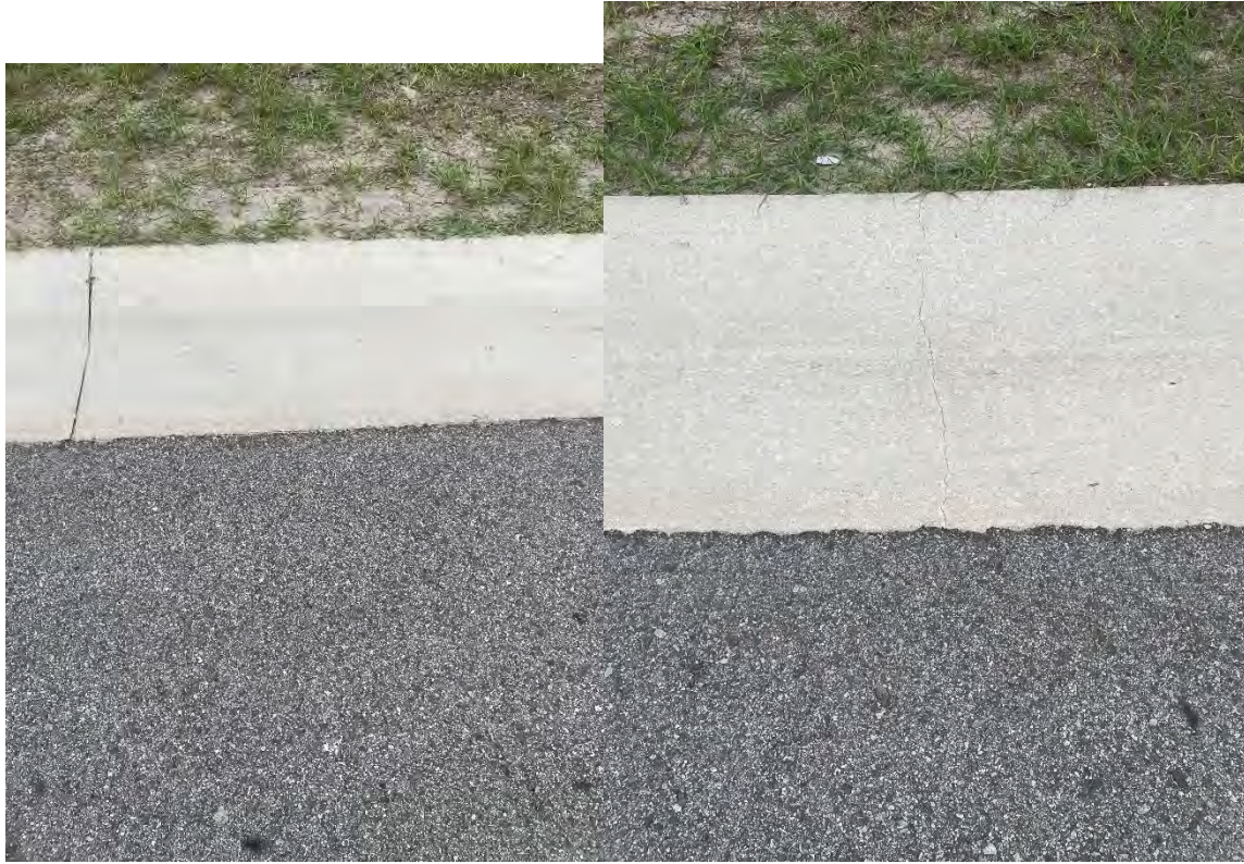
Gutter cracks across street from 13627 Seabridge
