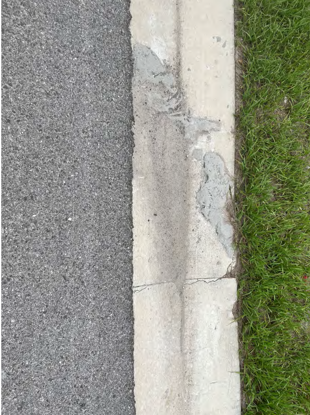
Gutter crack and excess concrete across from 13826 Moosehead
