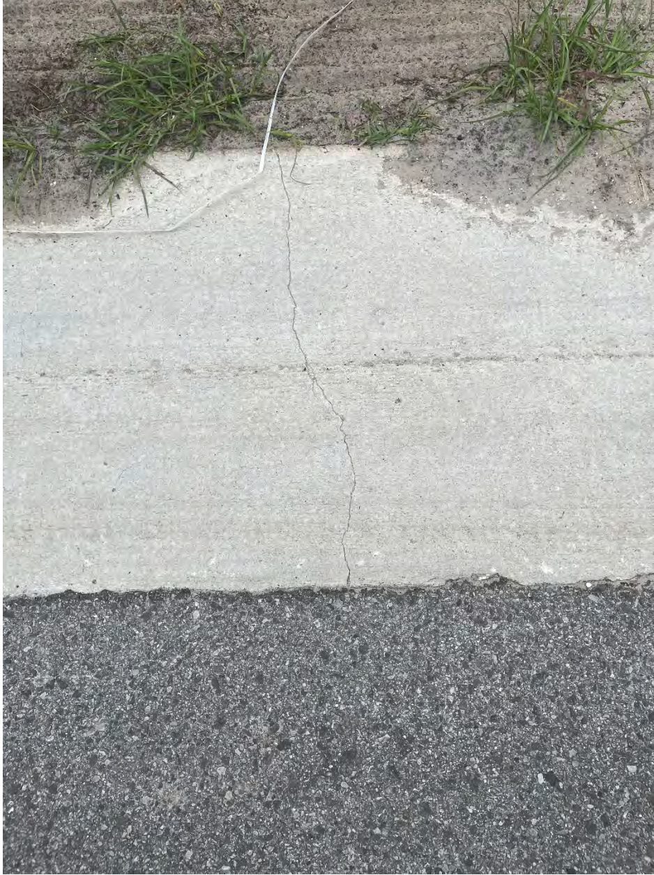
Gutter crack across street between 13539 and 13532 Seabridge
