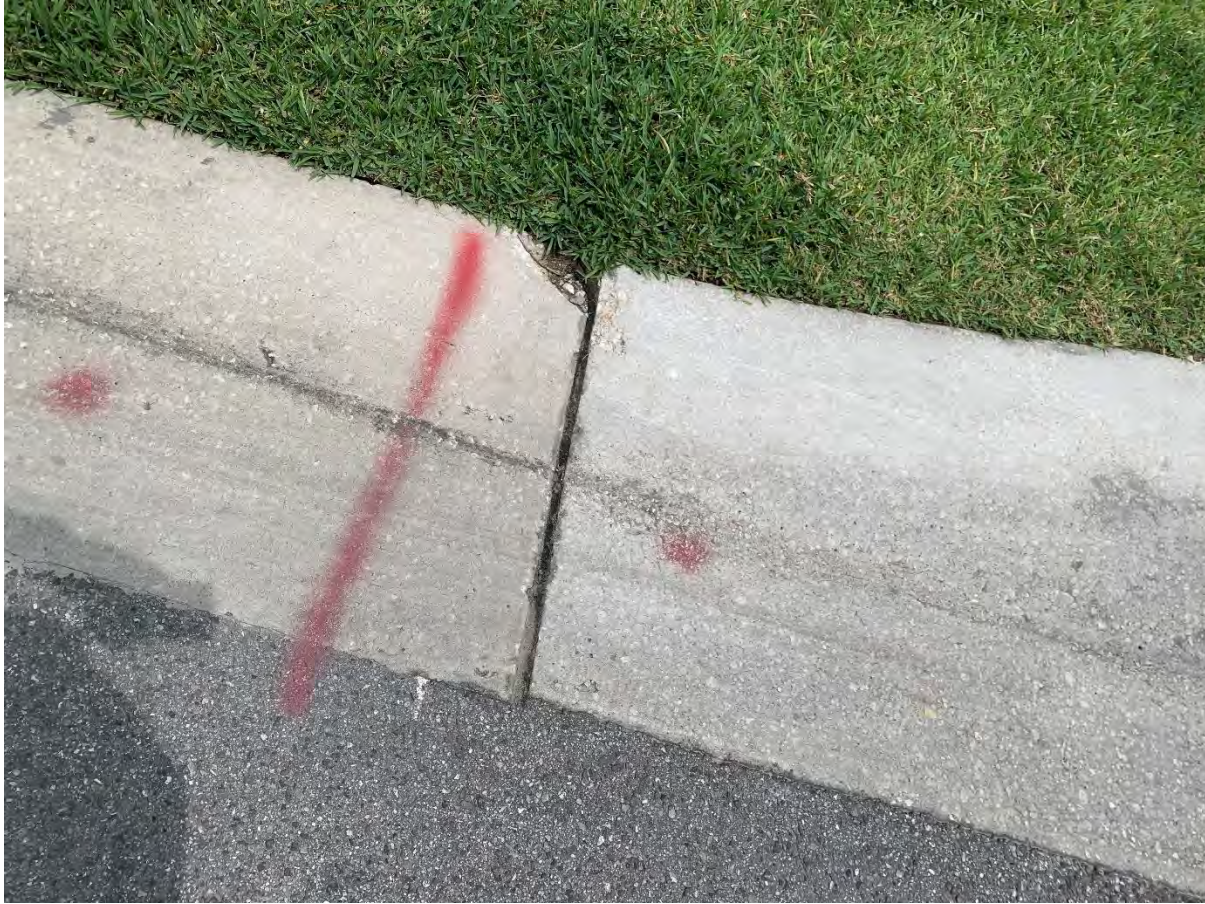
6 – Cracked guttering on Sea Bridge
