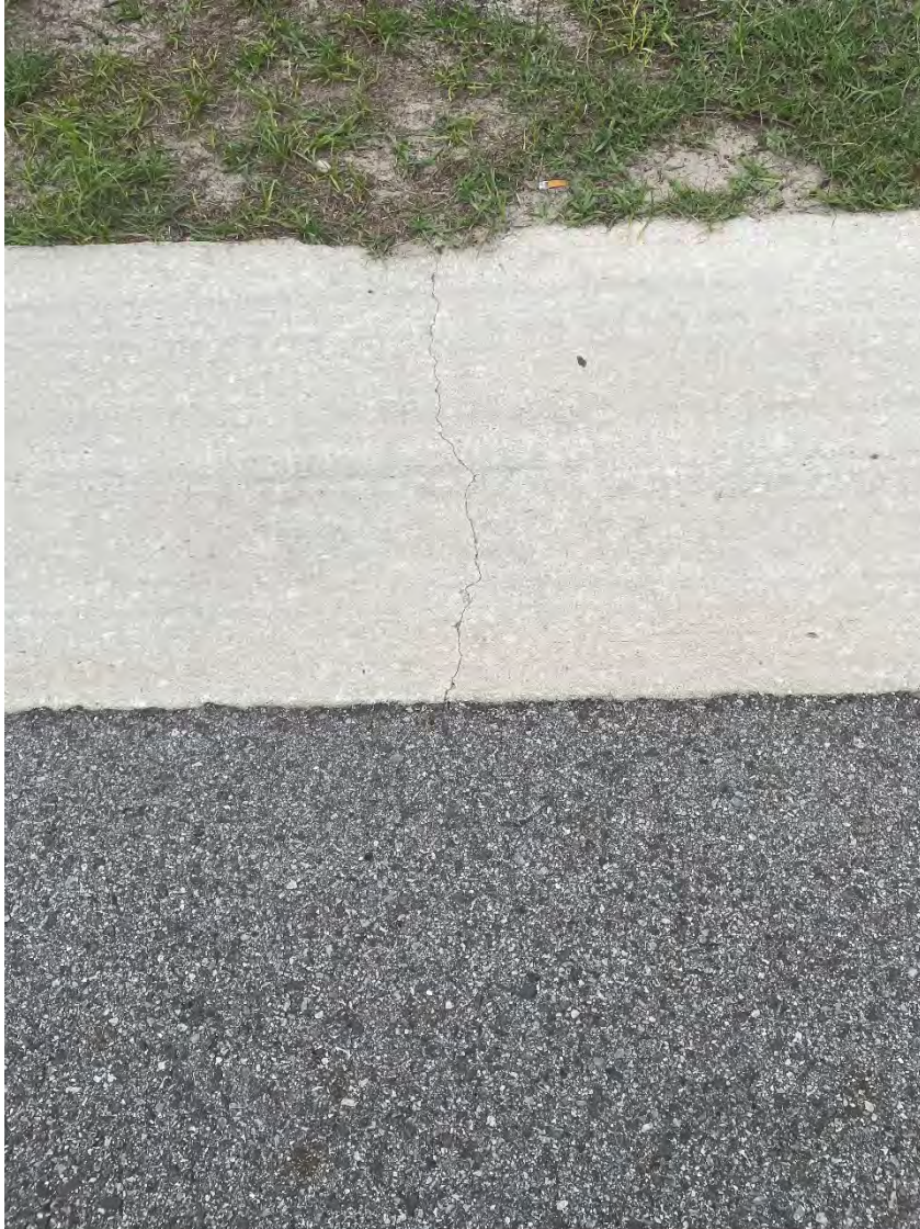
Gutter crack across street from 13611 Seabridge
