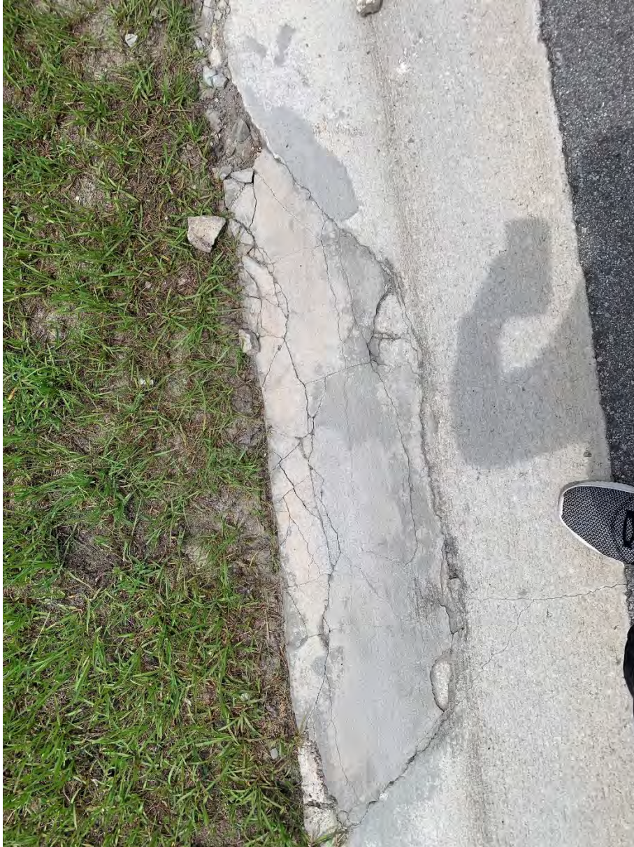
10- Gutter damage on Sea Bridge
